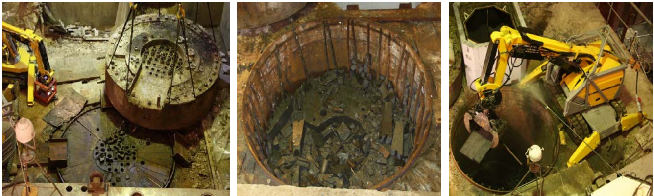
Fig.4 Unloading of graphite blocks.
